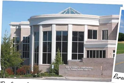
The County Courthouse
